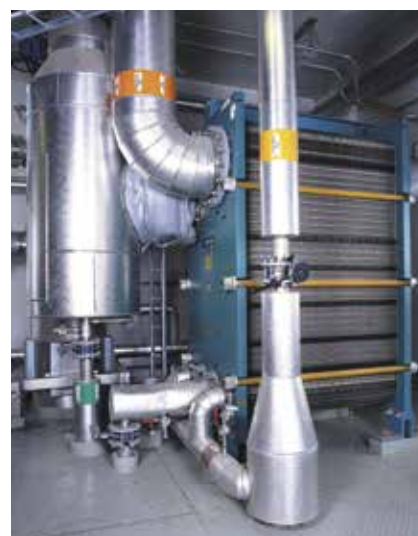
Ethanol condenser at The Absolut Company in Sweden. All the columns at The Absolut Company's Åhus distillery use Alfa Laval reboilers and condensers. The Alfa Laval units were chosen because of their compactness compared to corresponding shell-and-tube solutions.
