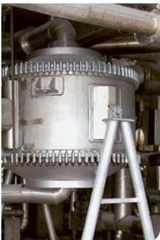
Spiral heat exchanger installation at the TOTAL refinery
