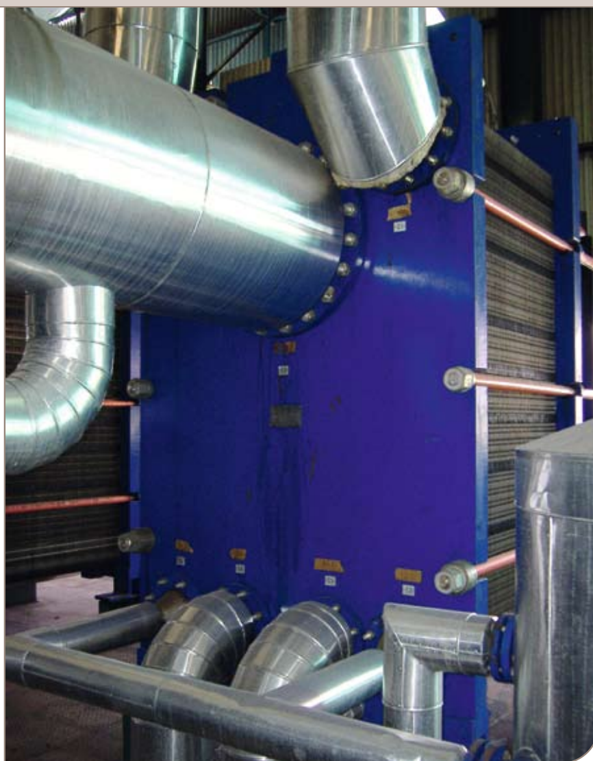
AlfaVap 600 plate evaporator in the sugar evaporation system installed by Alfa Laval at PT Angels Products.
