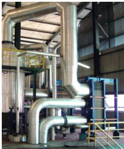
AlfaCond 600 surface condenser (bottom right) at PT Angels Products.
