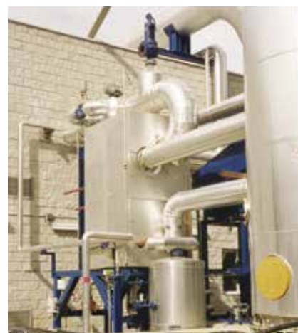
AlfaVap thermosiphon reboiler at Carboneco in Spain. The AlfaVap is used to boil 30% MEA at the bottom of the stripping column. The absorption-stripping system at Carboneco is used to recover carbon dioxide from a cogeneration plant. The system was built by the Danish contractor Union Engineering.
