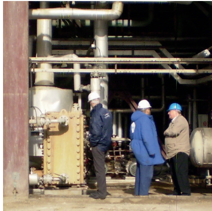
A Compabloc heat exchanger for preheating of Nitric acid.
