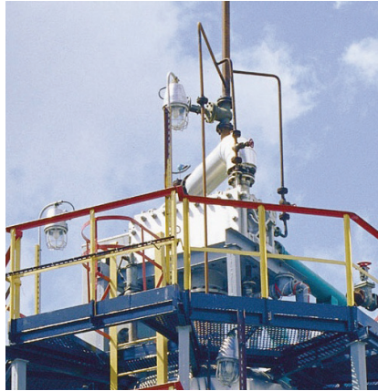
Compabloc reflux condenser mounted directly on the column
