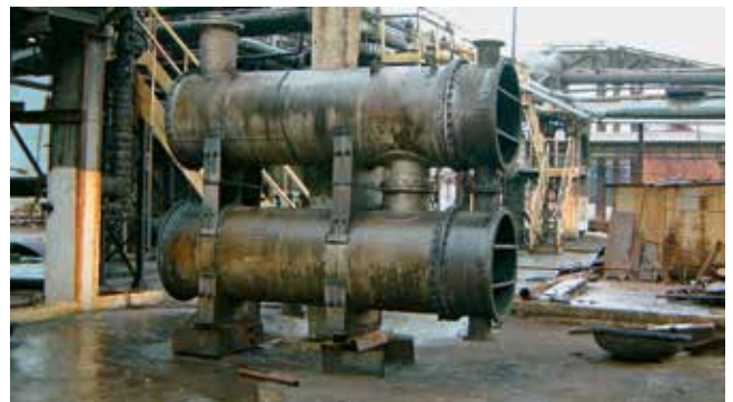
Two S&T heat exchangers replaced by one Compabloc resulting in better efficiency
