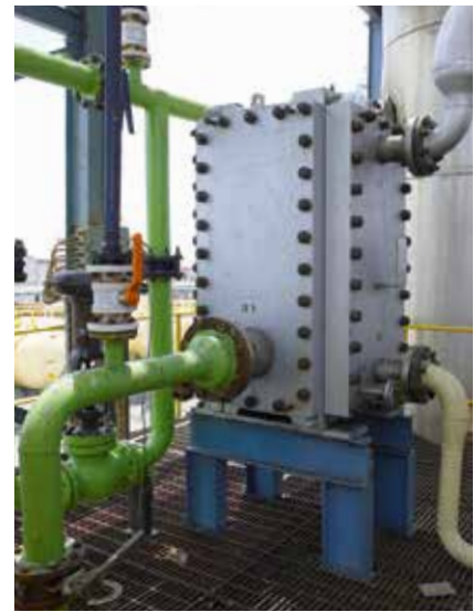
Compabloc compact heat exchangers replaced shell-and-tube units for heat recovery duties in the production of amines at BAL in India. A 40% reduction in steam consumption was achieved
