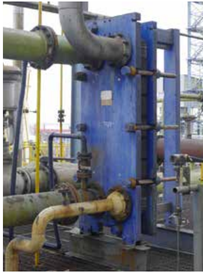
Compabloc compact heat exchangers replaced shell-and-tube units for heat recovery duties in the production of amines at BAL in India. A 40% reduction in steam consumption was achieved
